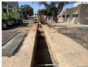
Bush Street Water Main Improvements
