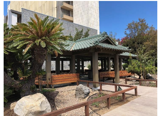
Civic Center Improvements: Pavilion Renovation
