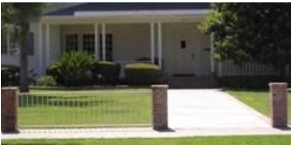
Wrought Iron Fence with Brick
