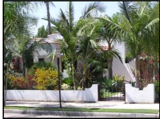
Example of Mission Revival-influenced fencing
