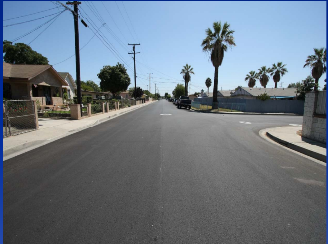
FINAL CIR PAVEMENT ON EVERGREEN AT FLORA
