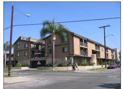
Ross Durant Apartments
