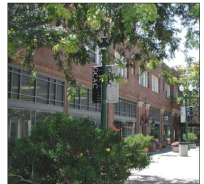
The City assisted in the restoration of the Grand Central Building for use by CSU Fullerton's Art Department. The property reopened in 1999 and is one of the major anchors of the Artists' Village in downtown Santa Ana.
