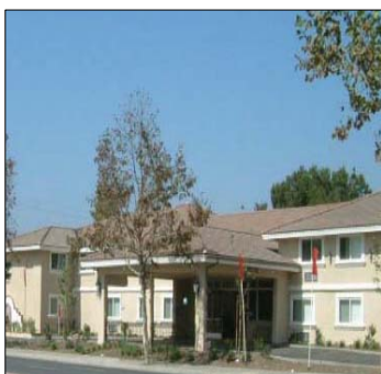
This motel was converted to 89 units of affordable senior housing with financial assistance from the Santa Ana Housing Authority, City of Santa Ana, and RDA.
