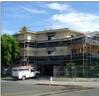
Sixth Street Apartments
